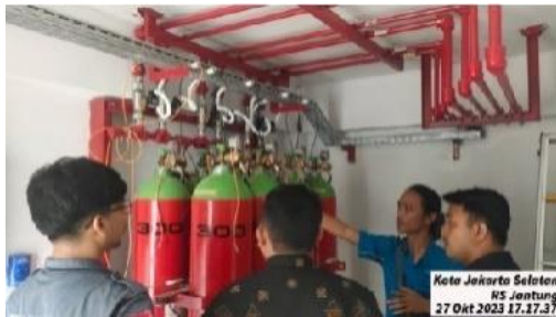
Inergen Fire Suppression Inergen System PT Jaya Kencana RS Jantung Kebayoran Baru
